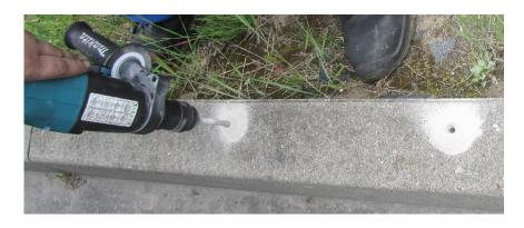
Screwing 3 MULTI-MONTI®-PLUS screws M10 X 140 mm per element. Connect the single elements with integrated connector pins.
