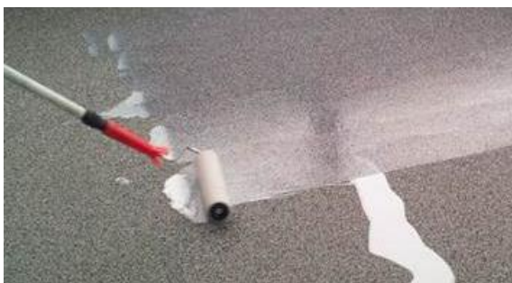
Image 3 and 4: application of the varnish
