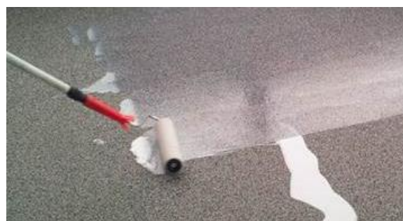
Image 3 and 4: application of the varnish
