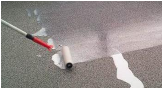
Image 3 and 4: application of the varnish
