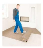
2. Place the underlay over the entire surface to be covered, laying it perpendicular to the subsequent laying direction of the floor finish. Leave the underlay in place for one day to allow dimensional relaxation and temperature equilibration.
