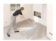
1. The substrate must be levelled and clean. If necessary use levelling compounds or primers. Check the usage instructions of the adhesive manufacturer for possible special procedures to follow over levelling compounds or primers if used.
