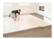
4. Fold back DAMTEC® black unito the middle of the room and glue the underlay to the substrate, observing the instructions of the adhesive and floor finish manufacturers.
