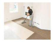
5. Put in DAMTEC® black uni without fold and rub and roll carefully.
