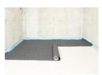
2. Place the underlay over the entire surface to be covered. Trim to size slightly larger than the surface covered. Leave the underlay in place for one day to allow dimensional relaxation and temperature equilibration.
