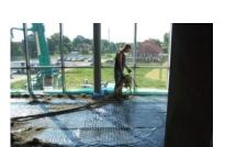
5. To avoid formation of sound conduction channels, be certain that screed cannot enter into the insulating underlay.
