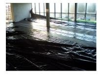
4. Cover underlay with PE membrane which should also cover the peripheral insulation strip and extend above the subsequent floor surface.
