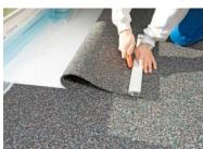
3. Use a regular carpet knife in conjunction with a steel straightedge for cutting to size.
