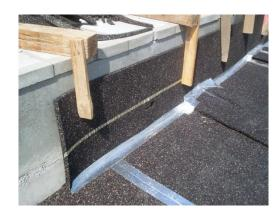
Vertical sections can be fixed using temporary mechanical devices (e.g. clamps, etc.) or with adhesive (Körapur 666 / Köracur TH 650). Ensure that no metal fixings are left in place that can cause sound bridging. The bonding of the side areas is over entire surface.
