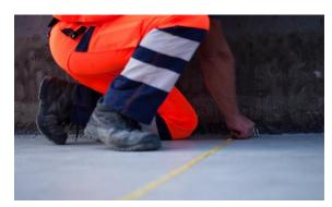
Especially at low temperatures, the sub-ballast mat should be rolled out on a flat surface about 1 hour before installation. Bulges on the front sides can be avoided.
