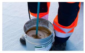
When installing the under ballast mat, they have to be glued on the substrate with a two-part polyurethane adhesive at certain points. The amount of adhesive should be about 25% substrate surface (for details see data sheet). The installation instructions of adhesive manufacturers have to be observed. The processing of the adhesive requires a dry and clean surface and a construction component- and air - temperature greater 10°C.
