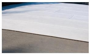
Joints have to be sealed using a special approved 75mm wide tape (type Gerband 613). While sealing the sub ballast mat has to be dry.
