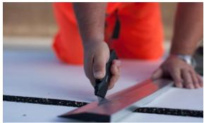
The mats must be laid at right angles to the track axis. The mats can be cut using a low speed sabre tooth timber saw or carpet knife and a steel straight edge. Before cutting ensure that the material is supported on an even hard surface.
