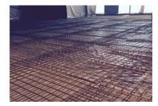
4. To avoid formation of sound conduction channels, be certain that screed cannot enter into the insulating underlay.
