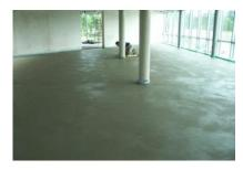
Install the screed or light weight cement. After finished installation start with floor finish. You can use other DAMTEC<sup>®</sup> products again for sound insulation.
