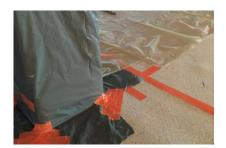
3. Cover underlay with PE membrane which should also cover the peripheral insulation strip and extend above the subsequent floor surface.
