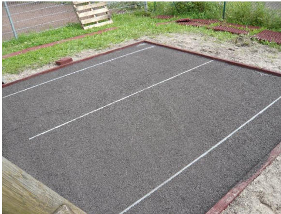
Levelling crushed sand/stone chippings
