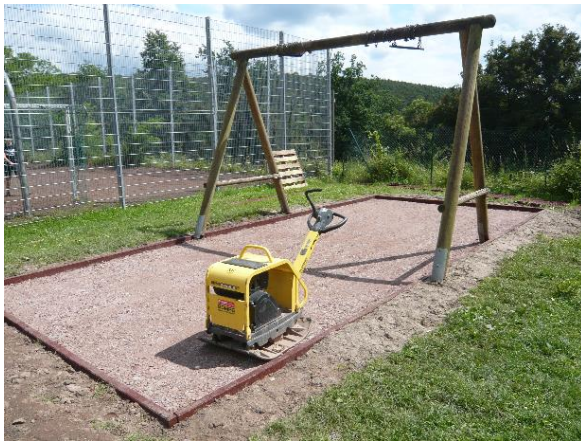
Crushed stones bed stable compacted
