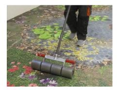
After a time interval of approx. 30-45 minutes (depending on the climatic conditions in the room), the covering must be rubbed again or rolled down with a cross-sectional roller. For the visual layer it is a sealer already factory provided applied.
