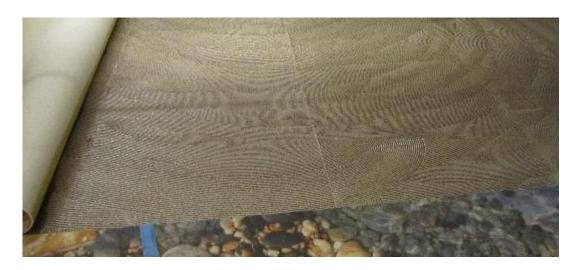
Every lane must press with the rub-on cork or pressure roller into the glue bed. To avoid glue on the layer material use crepe adhesive tape to save the joint areas. Glue spots on the layer must remove immediately.
