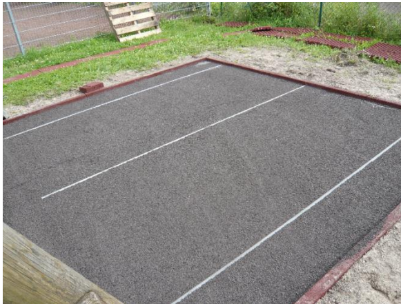
Levelling crushed sand/stone chippings
