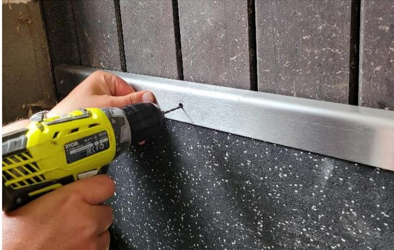
Depending on the existing box wall quality, wooden wall or concrete wall the appropriate countersunk screw is used and the tile is fixed with the stainless steel edging at a distance of 25 cm.
