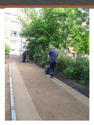
Evenly remove crushed sand - chippings mixture 0/5 mm, 0/8 mm and compact to a stable consistency.
