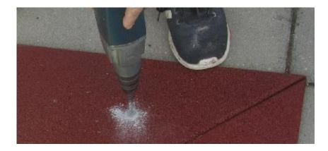
The screw head should be countersunk as deep as possible in the profile.
