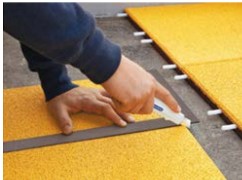
photo 5: Cut to size with a carpet knife
