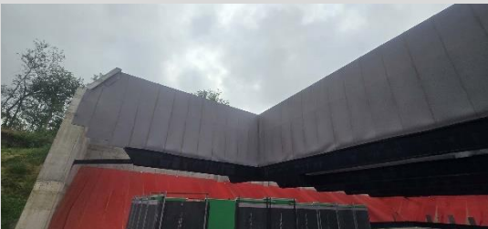
Fixing the mat to the wall with screw strips
