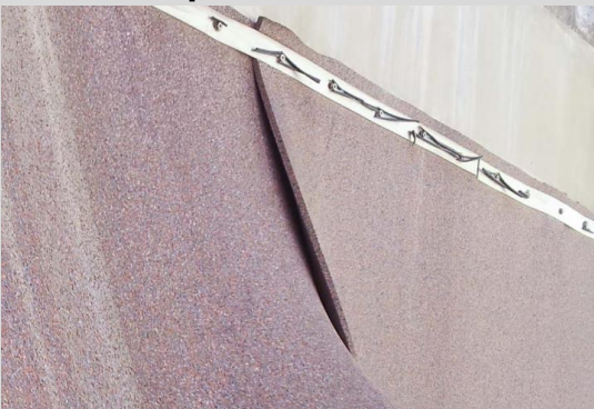
Fixing the mat to the wall with screw strips
