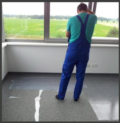
Create sections and apply the sealing liquid step by step from section to section.
