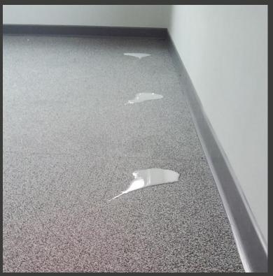
Spread the mixed sealer evenly onto the area that should be sealed, approx. 100g/m². Start at the edges of the room e.g.: walls and corners or in "difficult" areas.
