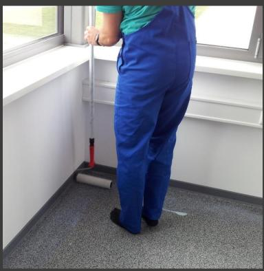
Spread the the sealing liquid at the edges and corners.
