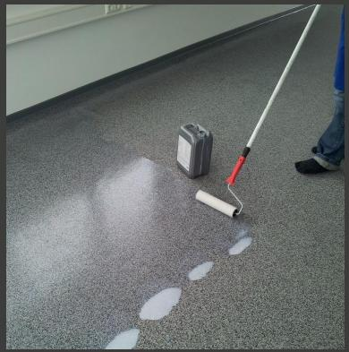
Once the walls and edges or "difficult" areas are finished, start the application of the sealer liquid on the rest of the floor.
