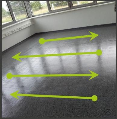
Roll out the sealer liquid in one direction (up and down) and then in a cross-wise direction (left and right) in one working step.
