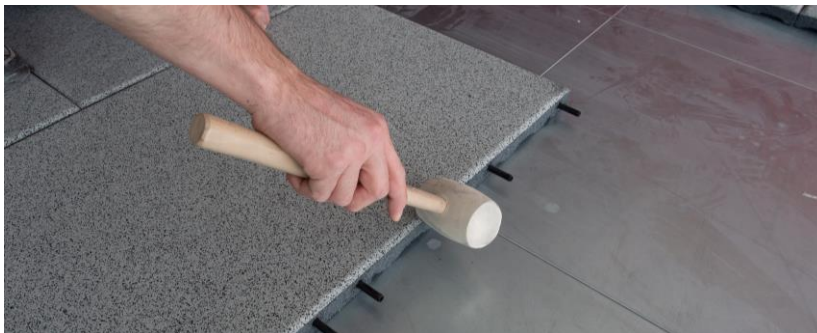
Closing the gaps with a hammer
