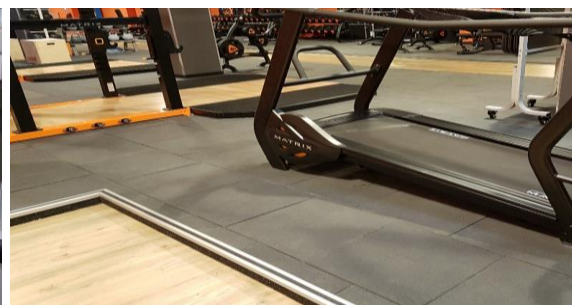
Perimeter step made by using a metal bar
