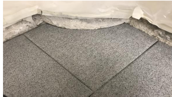
tiles can also be cut around curves
