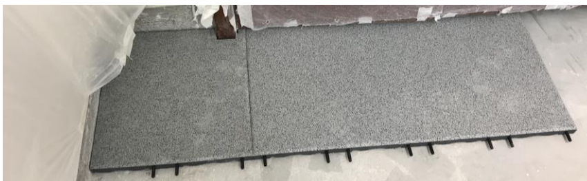
Installation of the tiles along a wall with the connector pins towards the next row
