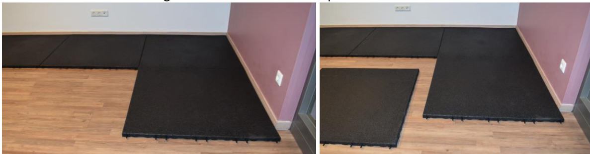
Installation of the tiles along a wall with the connector pins towards the next row
