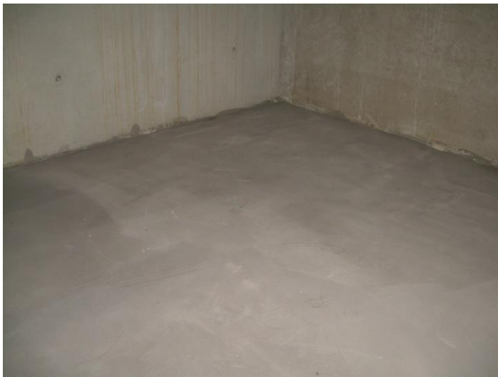
Even, suitable substrate made of poured screed
