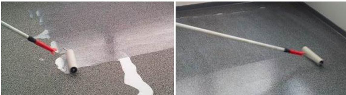
Applying of the coating
