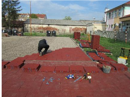
false installation in cross joints
