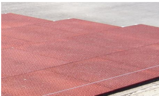
Installation of the tiles along an edging and chalk line
