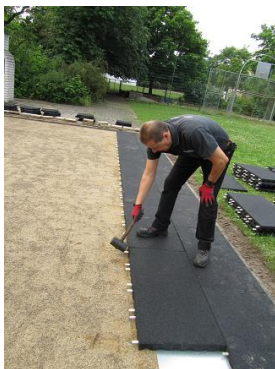
Using a hammer to close the gaps between the tiles
