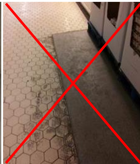
uneven, not suitable substrate
