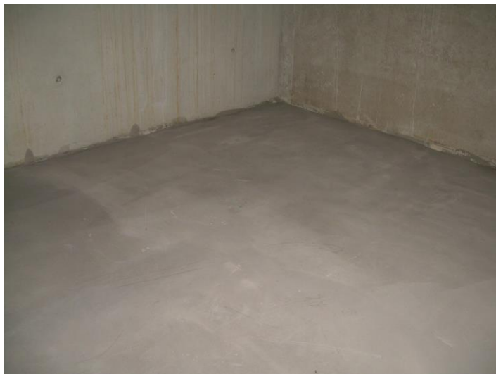
Even, suitable substrate made of poured screed
