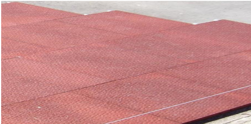
Installation of the tiles along an edging
