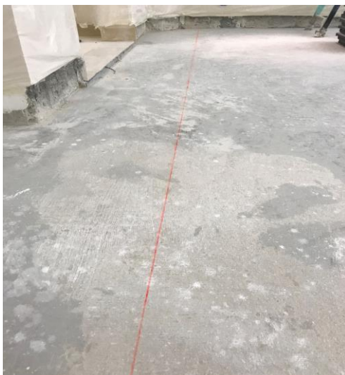
Creating chalk lines and laying the tiles along this line
