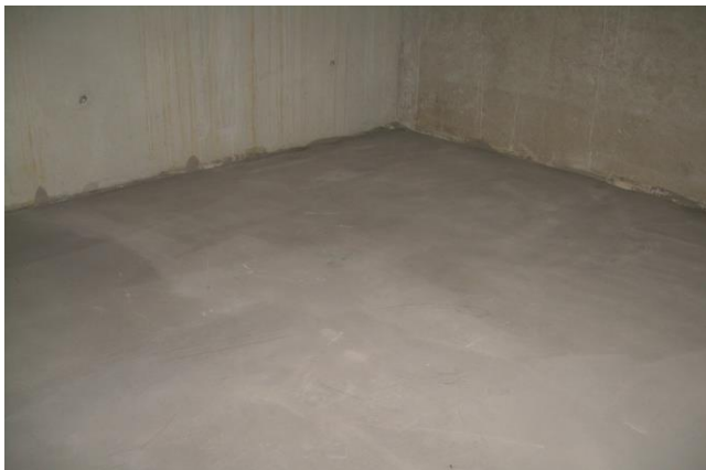
Even, suitable substrate made of poured screed
