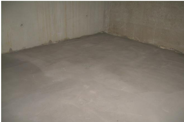
Even, suitable substrate made of poured screed
