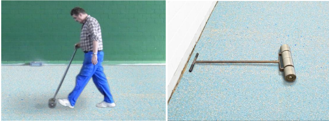
Scrolling of the floor with a pressure roller
