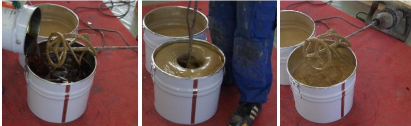
Mixing of the 2-component PU adhesive
