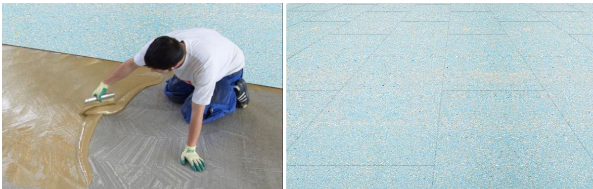
Adhesive application to clean substrate; roll out into the adhesive bed
