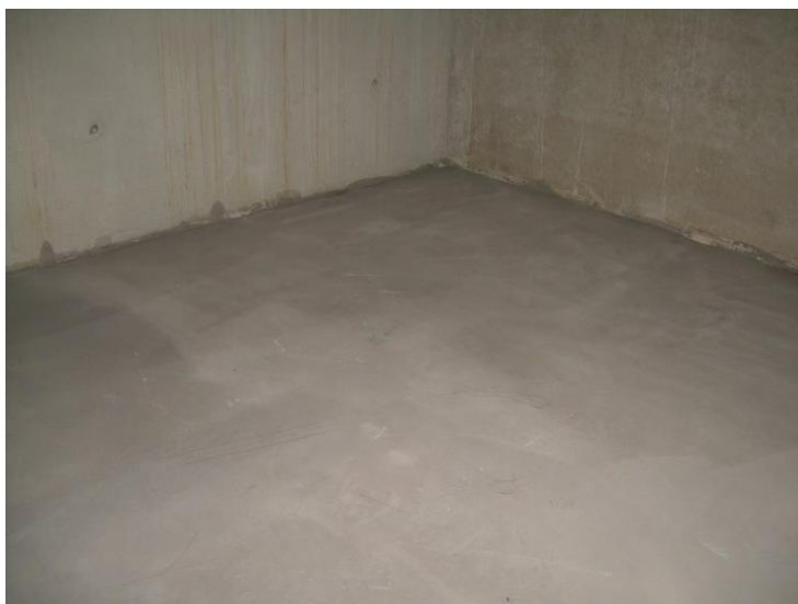
Even, suitable substrate made of poured screed
