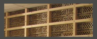
Our tiles are designed for installation without glue and should be installed in T-joints to the wooden slats. The tiles are connected to each other using the pre-installed connectors and fastened to the wooden battens with screws. All tiles can be cut to size with a jigsaw, industrial cutter or table saw.
