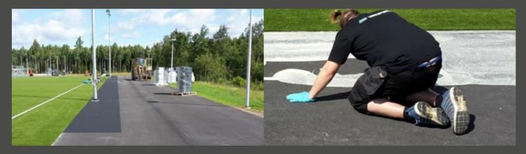
Always install the rolls with the underside (the side with the batch sticker) facing down and always in the same direction. Installation of the rolls should be with butted joints so that there are no gaps between the rolls.
